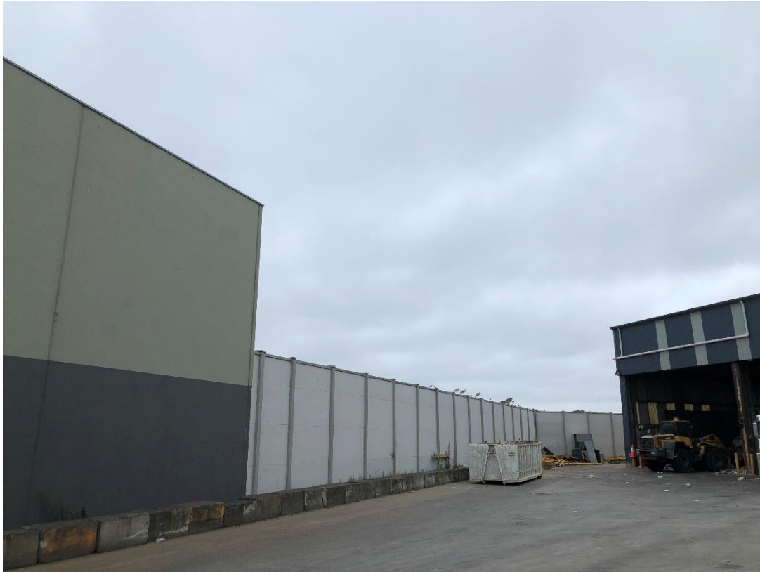
Figure 11 – Western edge of an adjoining building built to boundary which ties into the lower noise wall running along the boundary.
